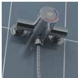
Exposed valve - bottom outlet
