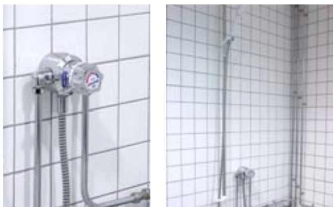
Less able shower facility with Meynell V8/3 thermostatic mixing valve with optional Special Needs Kit
