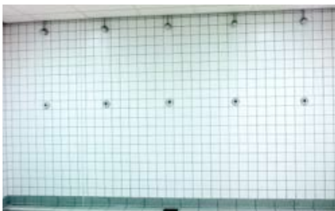
Group shower arrangement with Rada Pulse 129 no-touch sensors and VR125 vandal resistant shower heads
