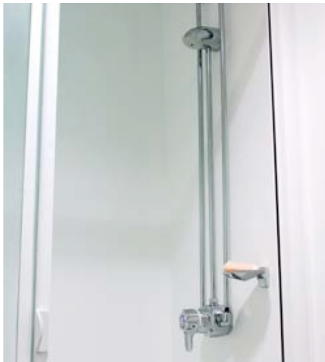
▲ Physiotherapist shower with Meynell V8/3L thermostatic mixing valve with Rada VR145 shower head.
