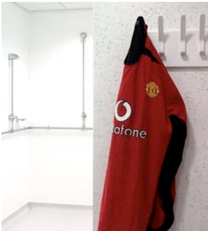
▲ Typical changing room arrangement with Rada 320c mixing valve (concealed in roof space), TF503 timed flow controls and VR145 shower heads ▼
