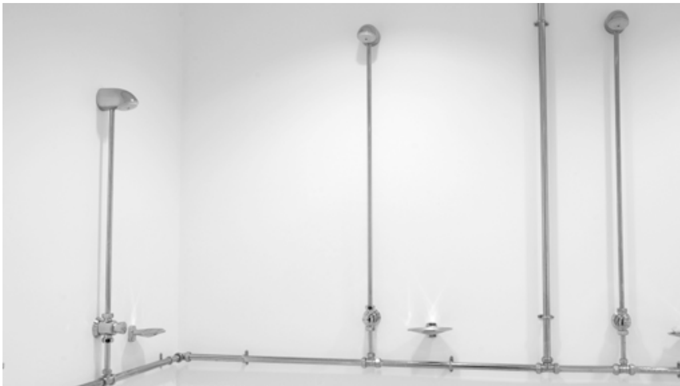
▲ Typical changing room arrangement with Rada 320c mixing valve (concealed in roof space), TF503 timed flow controls and VR145 shower heads ▼
